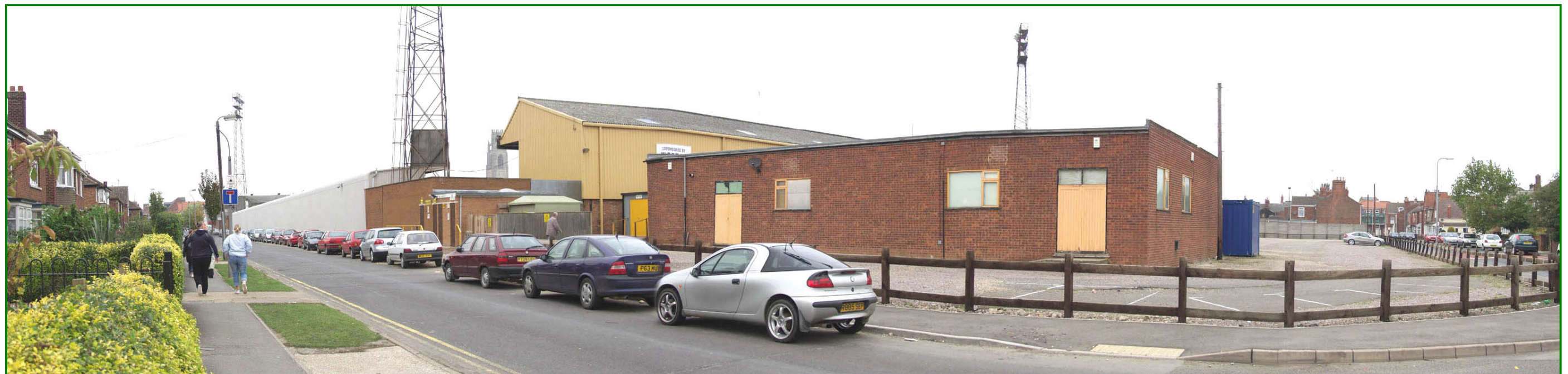
PLATE 6: View from corner of York Street and Spayne Road, looking north west towards the site.
